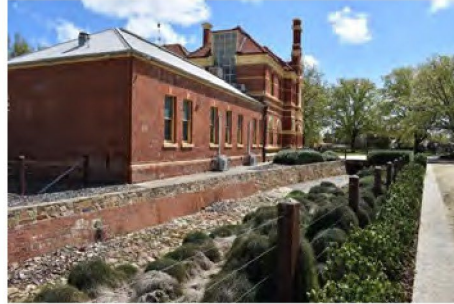
Figure 14. Oblique view of the Main Drain showing brick course and rubble construction.
