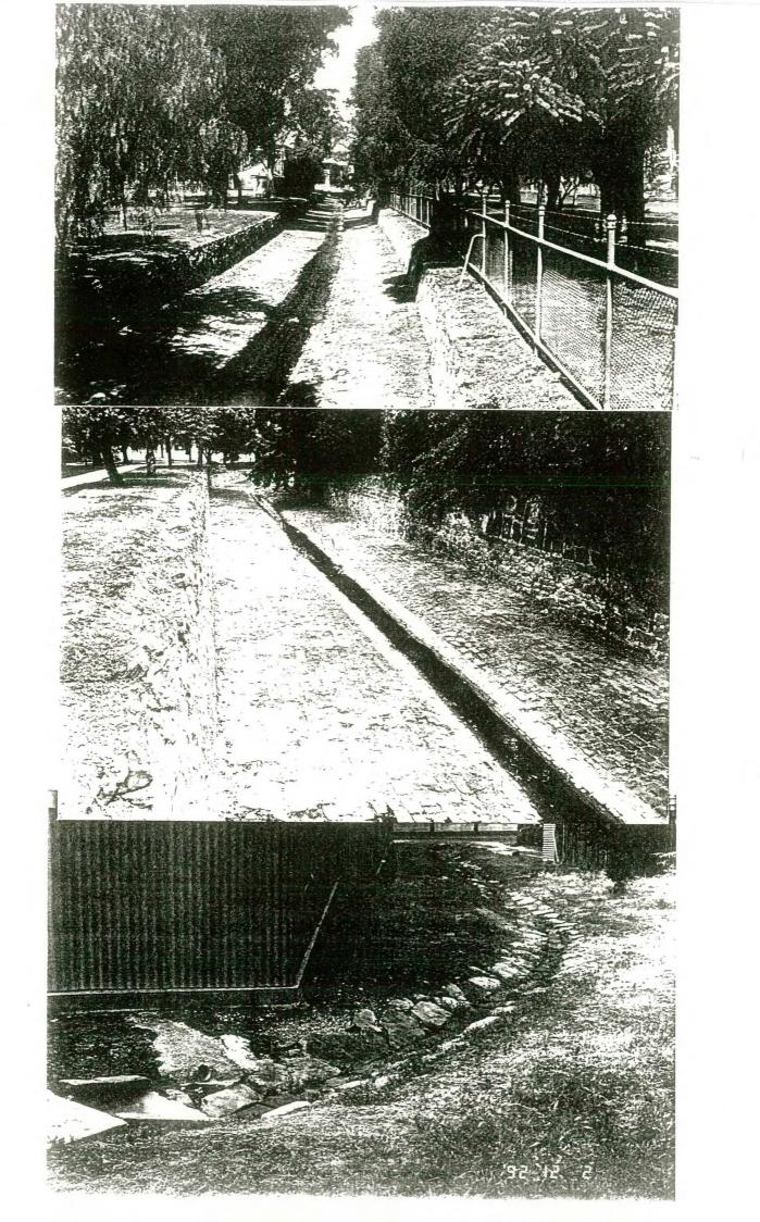
BLUESTONE LINED WATER CHANNEL SERVING FORMER CARISBROOK WATER SUPPLY DAM,
