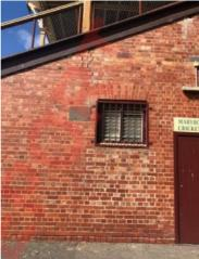
View of the northeast - corner where the timber post is leaning to the west. There is a visible lean to the west of the north-east cornet post. This is the site of previous alterations and settlement. The cause is unknown. Future maintenance is associated with repair of the masonry wall described below.
