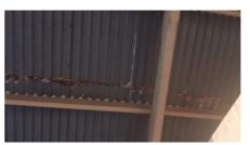
Repairs to corrugated iron roofing should be with galvanised corrugated iron to the original profile and thickness and using fixings to match the original. If possible, sheets in good condition should be retained and new rolled corrugated sheets to match existing profile, thickness and lengths. There are local manufacturers, ue of 9mm thick galvanized sheeting.
