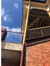
View of the rear walls mortar joints are loose and eroded.
