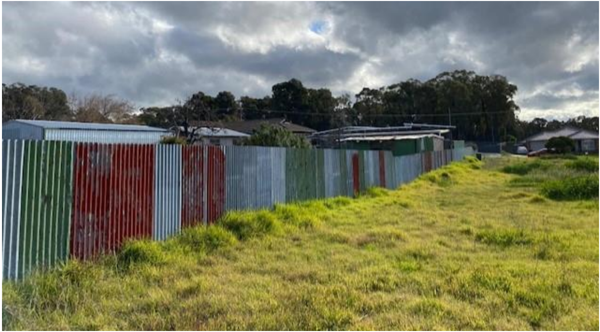
Internal western boundary fence
