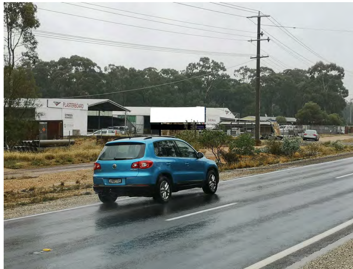
EXISTING PERSPECTIVE VIEW #02 - EASTBOUND TRAFFIC
