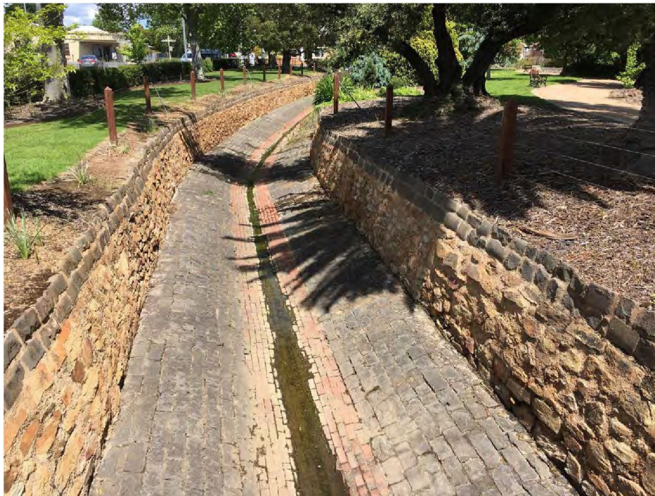
Figure 1. Main Drain within Phillips Gardens, initially built in 1873, then stone-lined in 1906.
