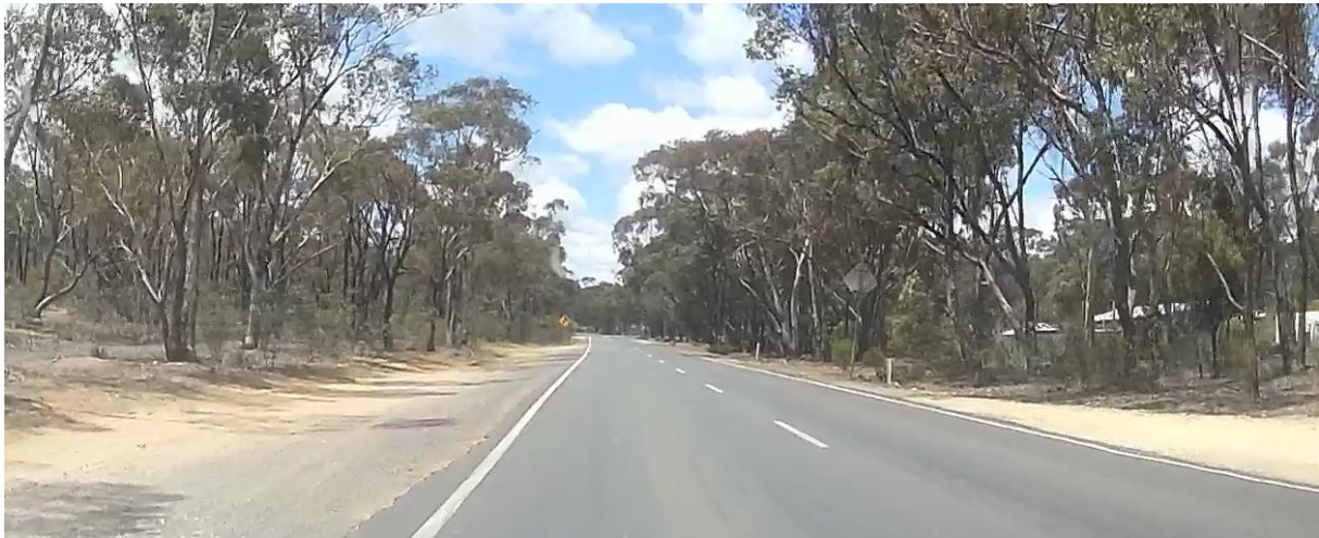
Figure 3.10: Phelan Road Facing South Toward Pyrenees Highway
