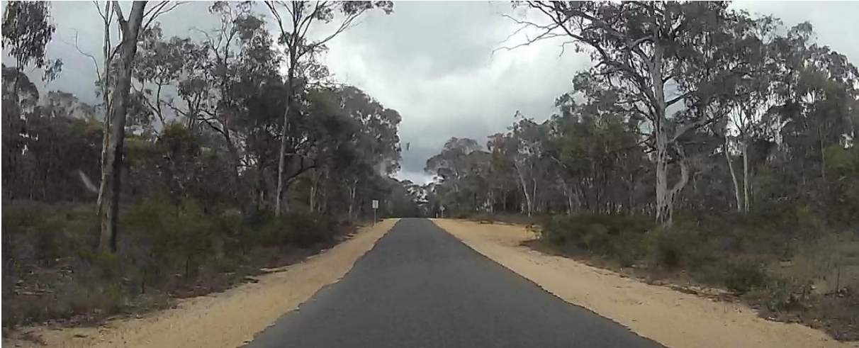
Figure 3.6: Old Avoca Road Facing South from Pyrenees Highway
