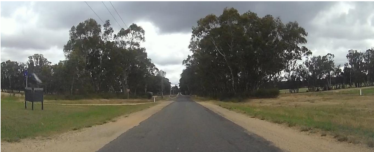
Figure 3.7: Old Avoca Road Facing North from Possum Gully Road
