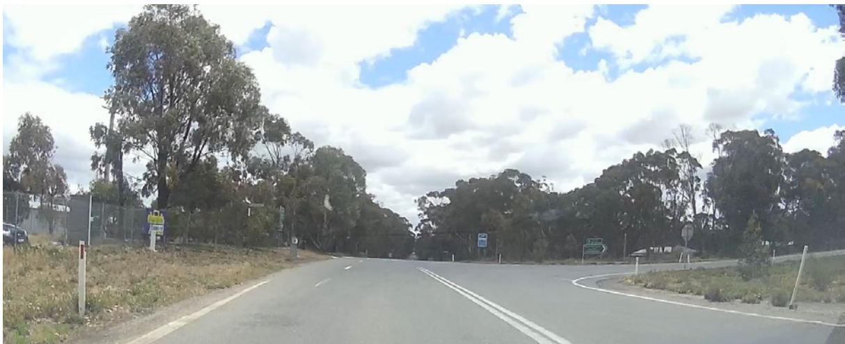
Figure 3.11: Phelan Road Facing North Towards Gladstone Street Intersection
