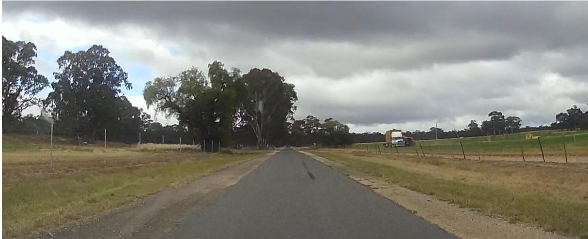
Figure 3.4: Possum Gully Road Facing South from Old Avoca Road Intersection
