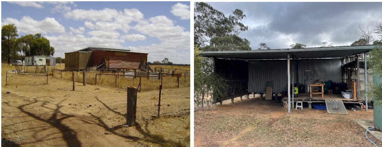
Figure 2 Left: Shearing shed in 2012 with the dwelling in the background facing SW Right: in 2025 where some walls have been removed to make way for a carport and work bench under the metal roof which was constructed not long before I purchased the property.
