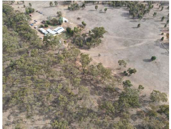
Fig.25 Looking over the woodland vegetation to the south of the development site.
