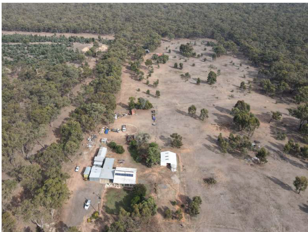
Fig.3 View of the property and existing infrastructure.
