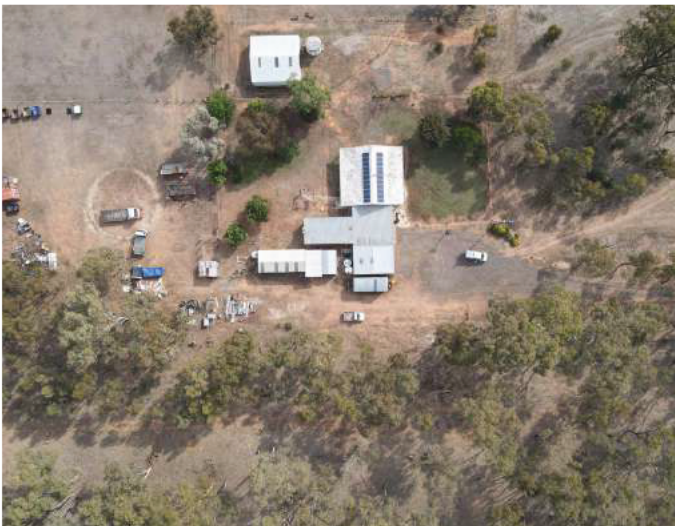
Fig.26 Looking from directly above the development site.
