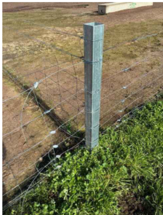
GALVANISED STEEL POSTS IN CONCRETE H: 1.2m GALVANISED WIRE MESH H: 1.15m
