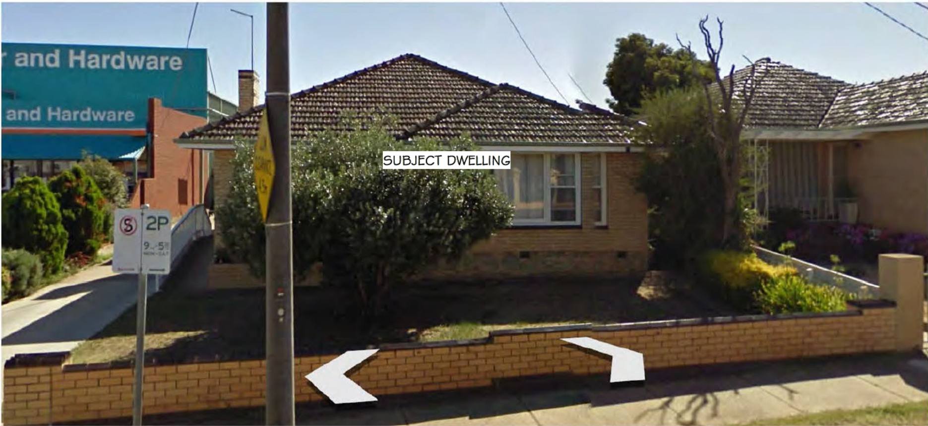
DWELLING TO BE DEMOLISHED TUAGGRA STREET VIEW
