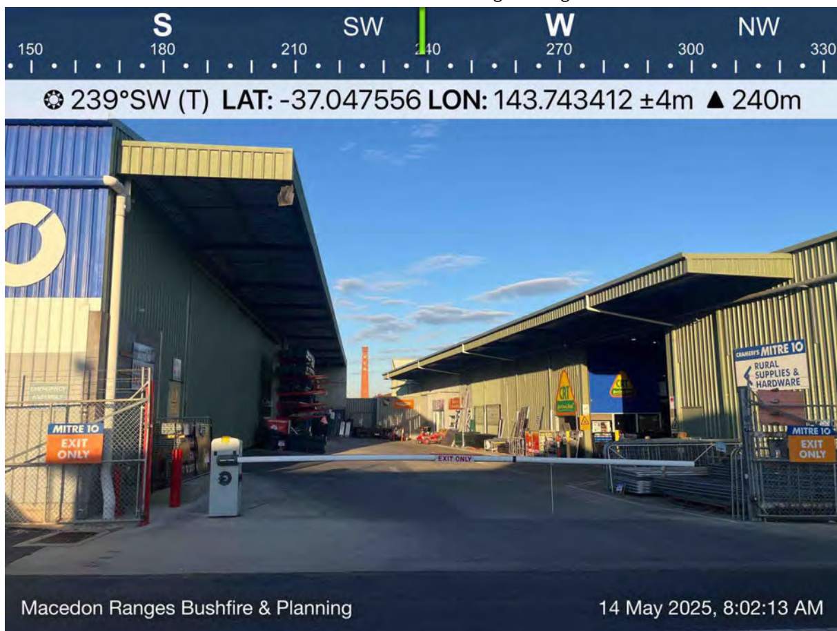
Exit of drive through to Crameri Lane
