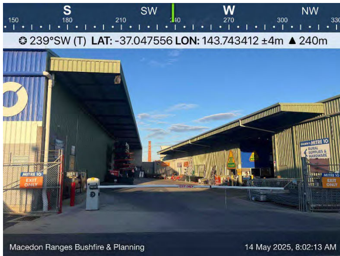
Exit of drive through associated with Mitre 10
