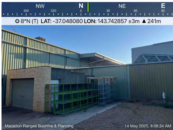
Outbuilding of dwelling at 16 Tuaggra to be demolished
