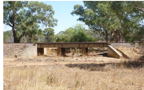
19 – Local drainage railway crossing
