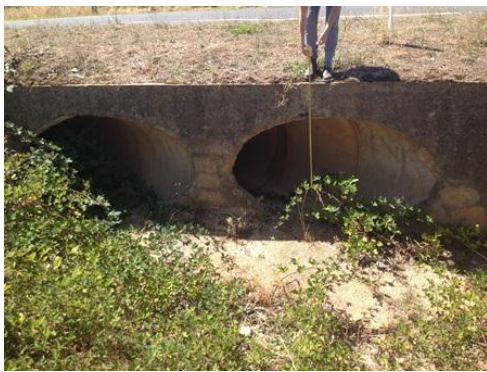
17 – Local drainage at Dunolly Rd
