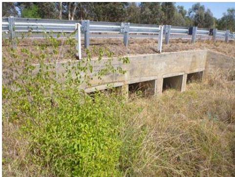
06 – Local drainage at Dunolly-Moliagul Rd
