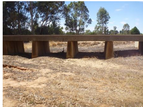
05 – Local drainage railway crossing
