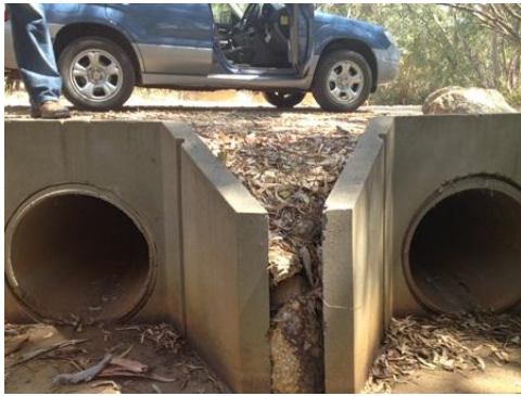
15 – Burnt Creek at Maude St
