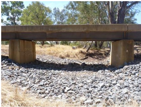
08 – Burnt Creek railway crossing
