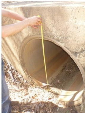
01 – Burnt Creek at Burnt Creek Lane
