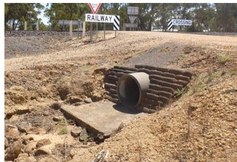
07 – Local drainage at Hospital Street
