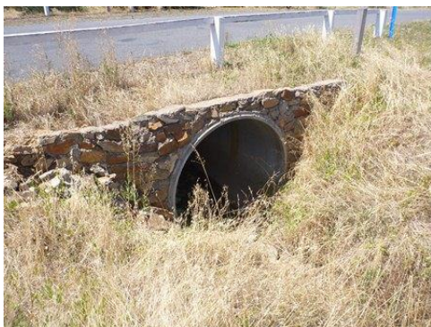
10 – Local drainage at McKinnon St
