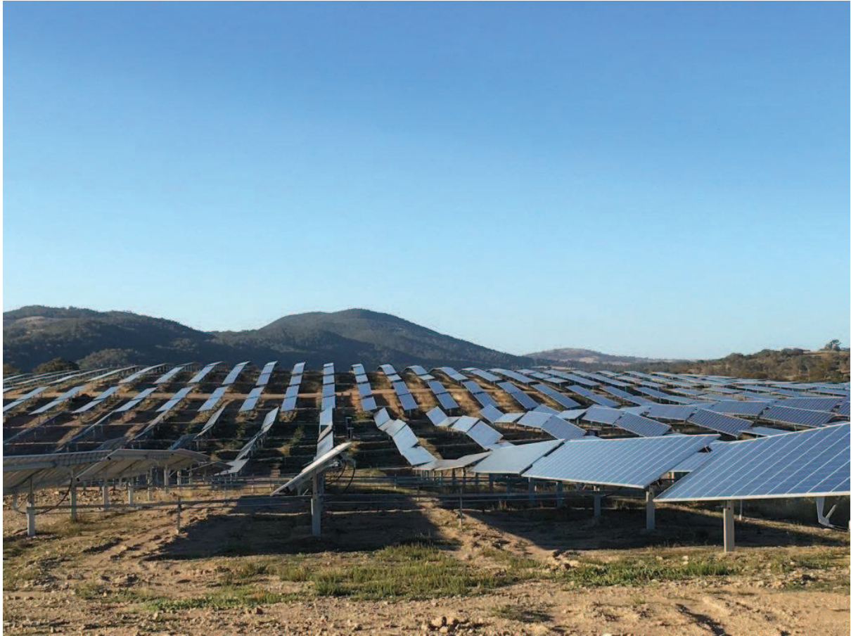
Figure 14: Example of Solar PV Arrays
