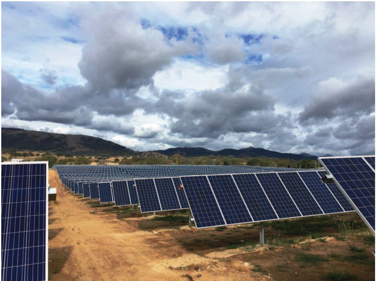
Figure 13: Example of Single Axis Solar PV Arrays
