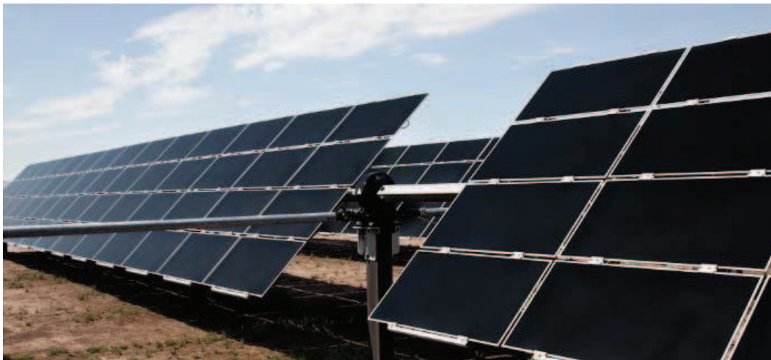
Photo 1. Example of a typical frameless solar array 6
