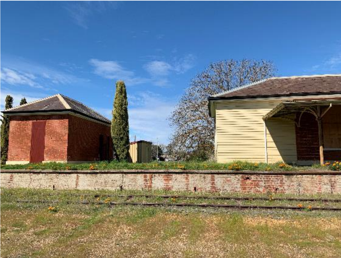
Photo 9 – Abandoned Carisbrook Train Station
