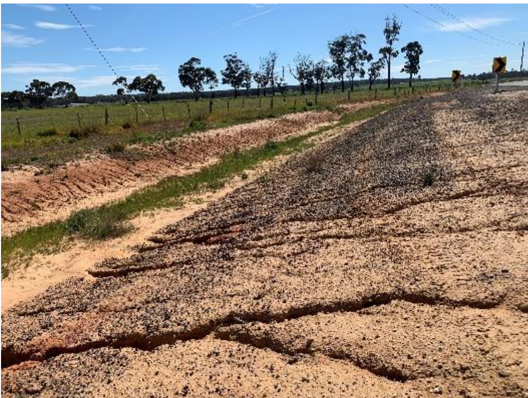
Photo 8 – Behind photo 7 looking south. (Stage three (3) of proposal)
