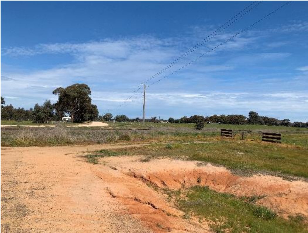
Photo 7 - Location of proposed culvert under railway line (Stage three (3) of proposal)
