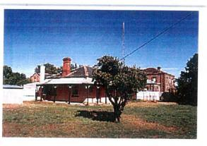
building retains its timber double hung windows. There is a later unsympathetic skillion roof addition to the rear of the building and a number of later sheds on the site.
