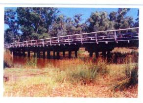
increasing expense of large and durable bridge timbers, and the greatly increased trafficloading requirements of the post-war reconstruction era, the building of large all-timberbeam bridges fell off drastically.
