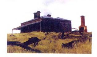
The stables building has a steeply pitched hipped roof clad in corrugated steel and only has a small opening near the eaves line in the wall facing into the courtyard. At one end it has a very wide opening with a timber lintel just under the eaves. Again the gutter is missing.
