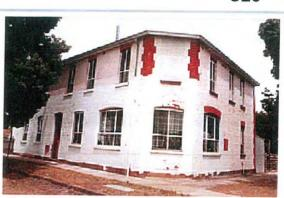
Externally the building is substantially intact in that it retains its basic form, face brick wall material (although painted) most window and door openings. Integrity
