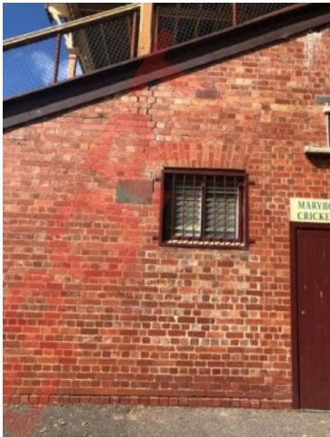
View of the northeast - corner where the timber post is leaning to the west. There is a visible lean to the west of the north-east corner post. This is the site of previous alterations and settlement. The cause is unknown. Future maintenance is associated with repair of the masonry wall described below.
