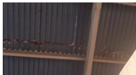
Repairs to corrugated iron roofing should be with galvanised corrugated iron to the original profile and thickness and using fixings to match the original. If possible, sheets in good condition should be retained and new rolled corrugated sheets to match existing profile, thickness and lengths. There are local manufacturers, use of 9mm thick galvanized sheeting.
