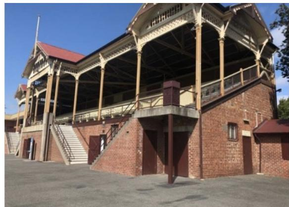
The Grandstand in 2021, replaced enclosed brick stairs and replaced original balustrade and altered fenestration at ground level.
