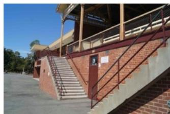
View of the replaced brick and concrete stairway, new doorways and replaced timber balustrading.
