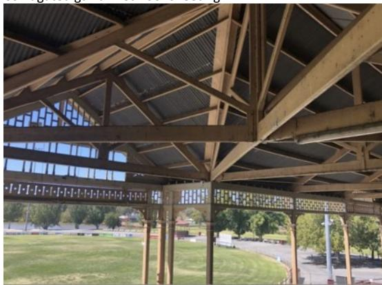
Structural timber, series of roof trusses support the main hip and five gables.
