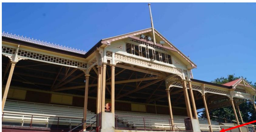
It is recommended that all missing decorative timber detailing is reinstated. Loose timber decorative details have been removed and stored at the Council depot for safe keeping and safety. I:I scale dimensioned sketches should be prepared for reconstruction and replacement exactly like for like. This includes replacing the balustrade.
