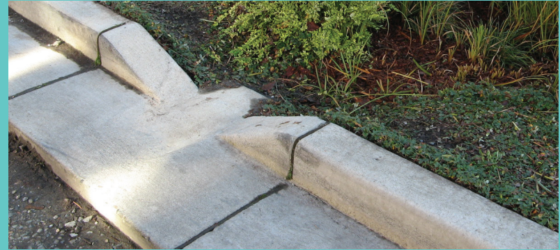
Example of dropped kerb to facilitate passive irrigation
